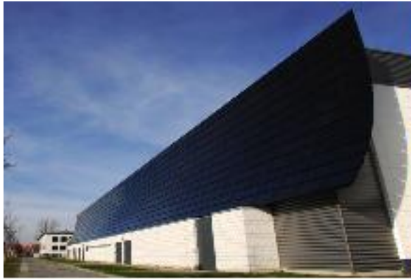
Left: building integrated PV fasade (location: Ferdinand Braun Institute, Berlin, Germany).
