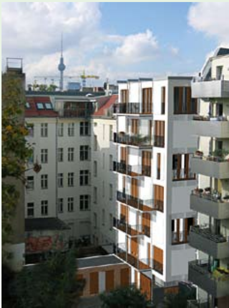
Figure 5: Seven-storey wooden apartment block in Berlin-Pankow (completion 2008). Source: Kaden + Klingbeil Architekten, www.kaden-klingbeil.de
